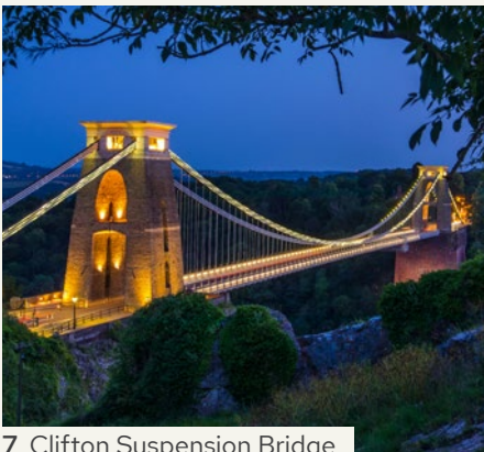
7 Clifton Suspension Bridge
